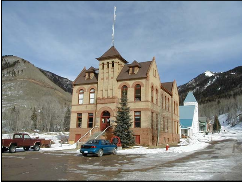
The Rico Town Hall is located in the historic Dolores County Courthouse, constructed in 1891. This building has undergone an extensive Phase I exterior restoration which involved replacing deteriorated masonry, repointing all masonry, and replacing the front steps. Phase II of restoration is planned to begin in 2004.
