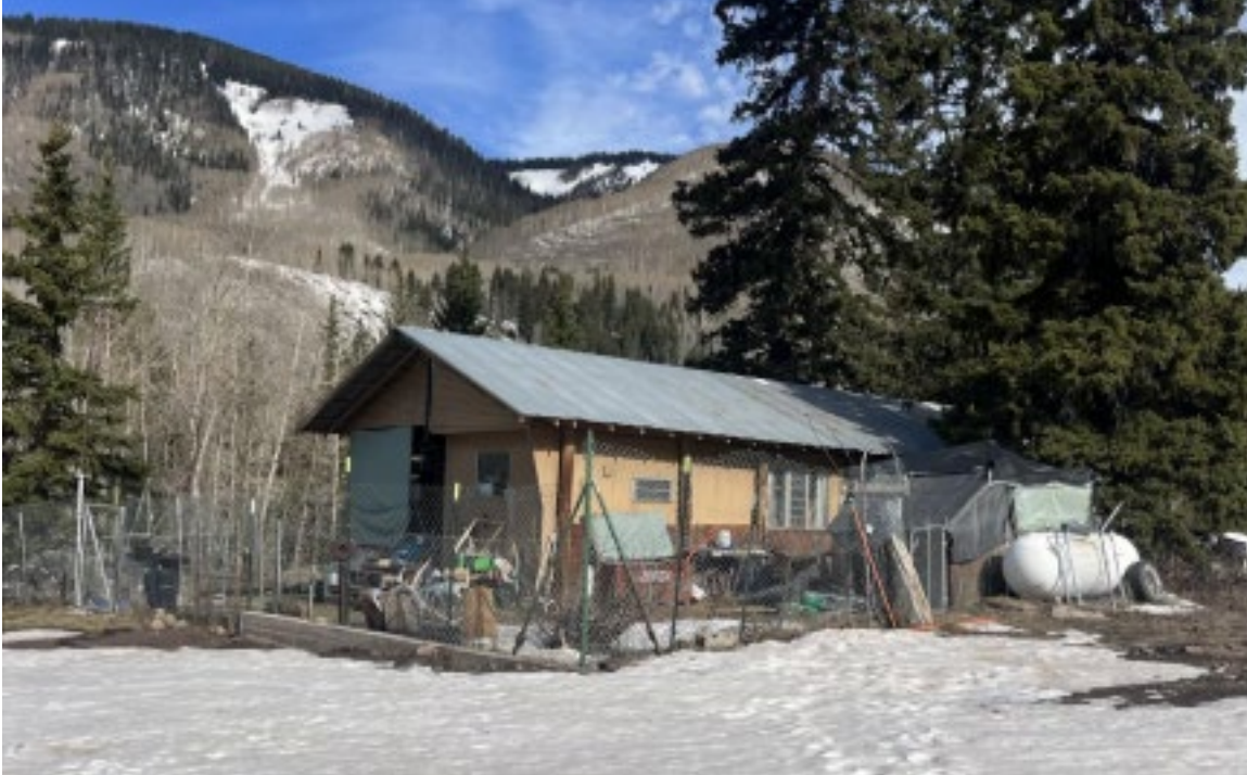
Trailer located on a portion of lots 39 and 40, Block 2
