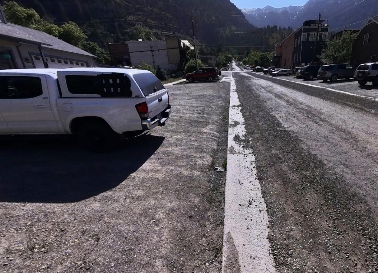
Figure 2 - Erosion Alongside Waterway, Ouray Colorado
