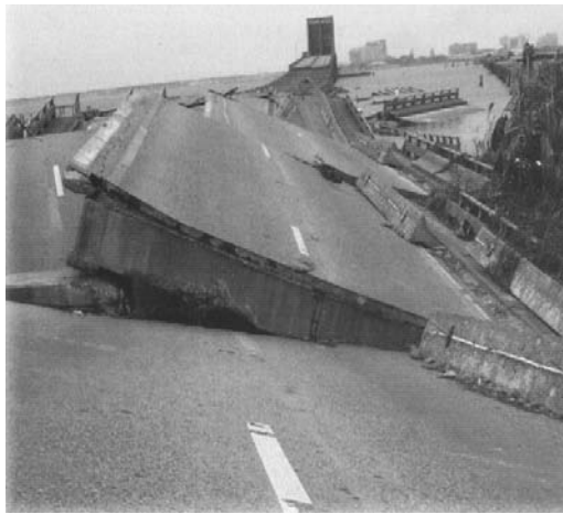
Biloxi, Mississippi, USA. On Aug 30, 2005, the Louisiana and Mississippi coasts were hit by a category 4 storm with maximum winds at 140 mph. This bridge was no match for Hurricane Katrina. This vital link connecting Biloxi to Pascagoula was swept 30 feet off its pylons and cast into the sea. The bridge remains closed eight months after the storm.
