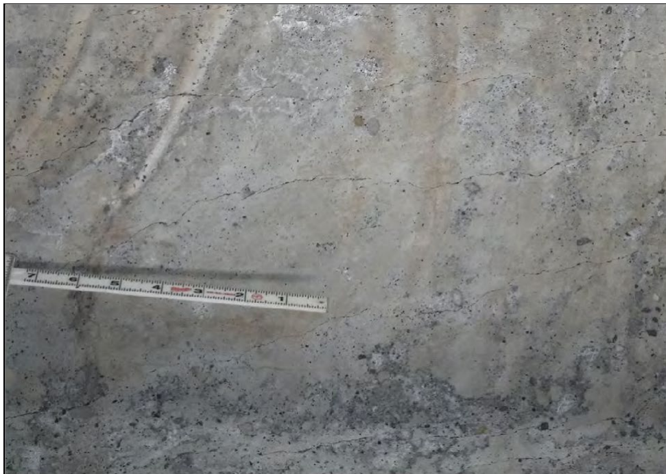
Longitudinal cracks in soffit of Bay C
