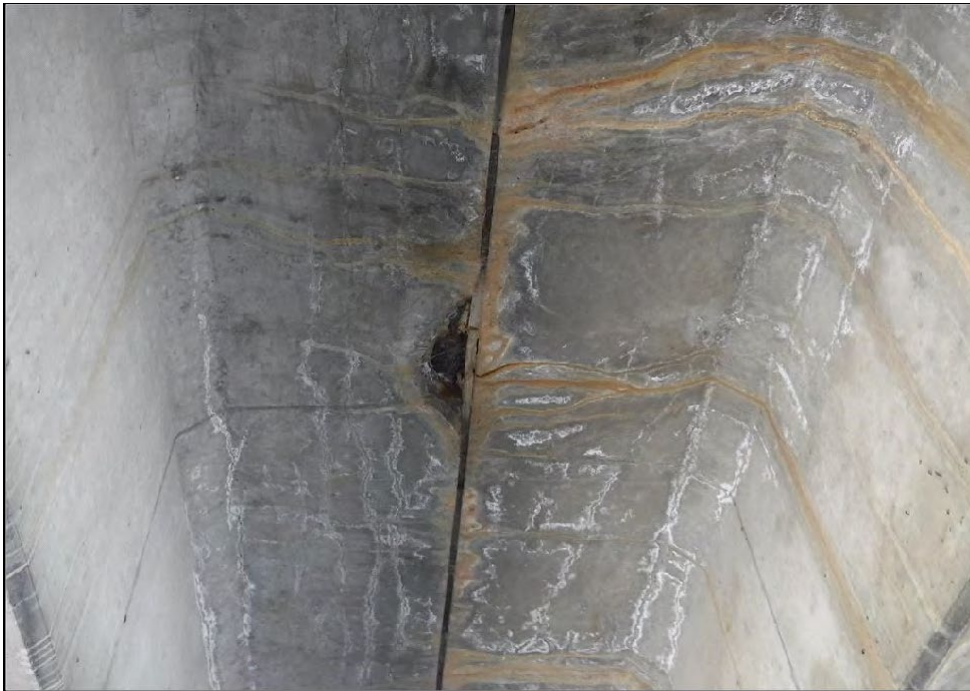
Spall in Girder A top flange near Abutment 1
