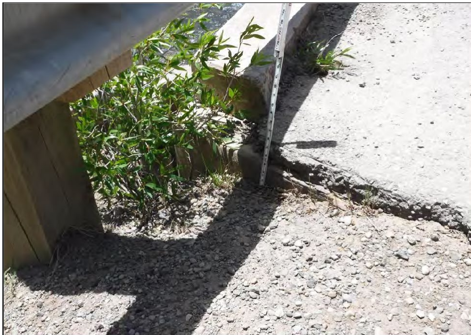
Erosion at northeast corner of deck
