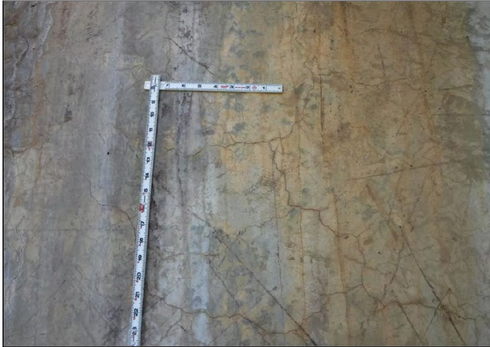
Map cracking in Abutment 2
