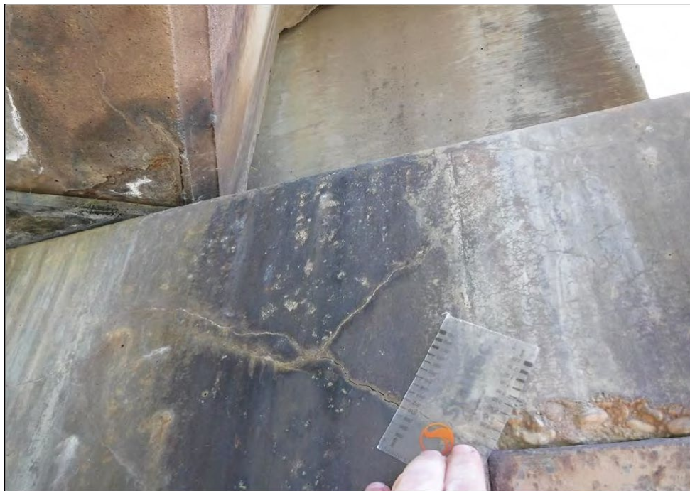
Cracking in pier cap under Girder D at Abutment 2
