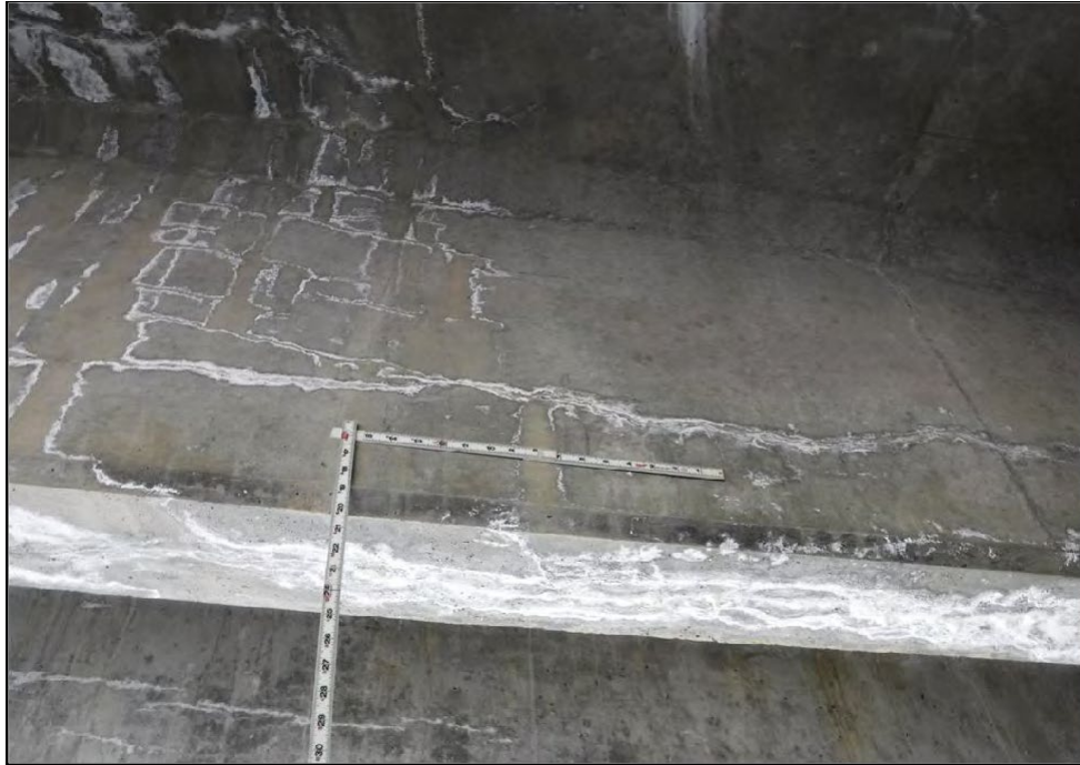
Horizontal crack with efflorescence in Girder C near Abutment 1
