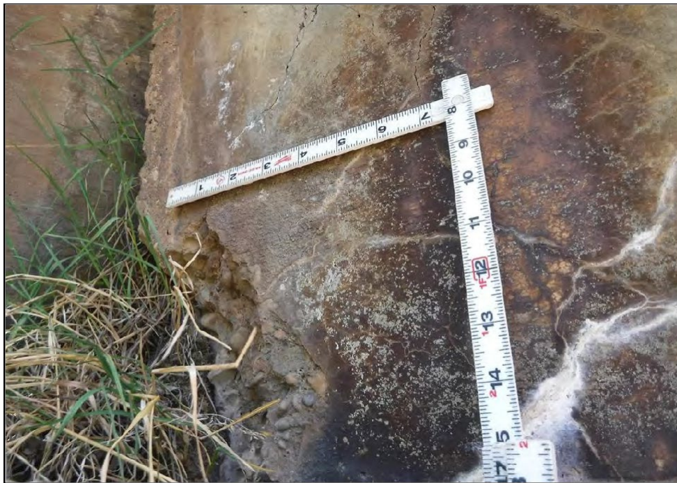
Spall in Girder D at Abutment 1
