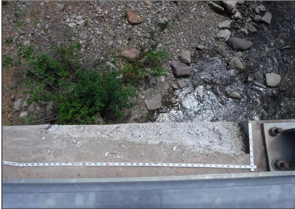
Spall in east curb
