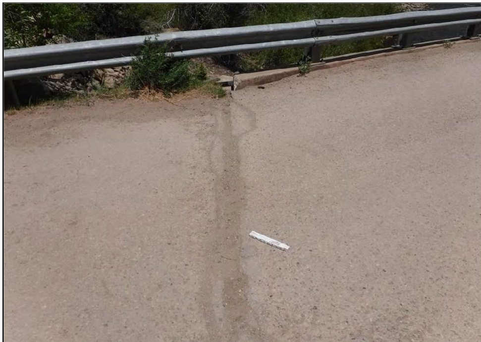
Transverse crack in asphalt over Abutment 1
