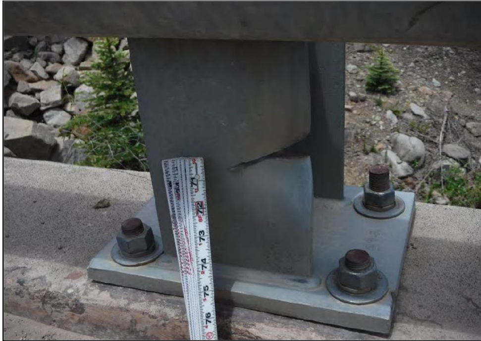
Tear in west bridge rail post
