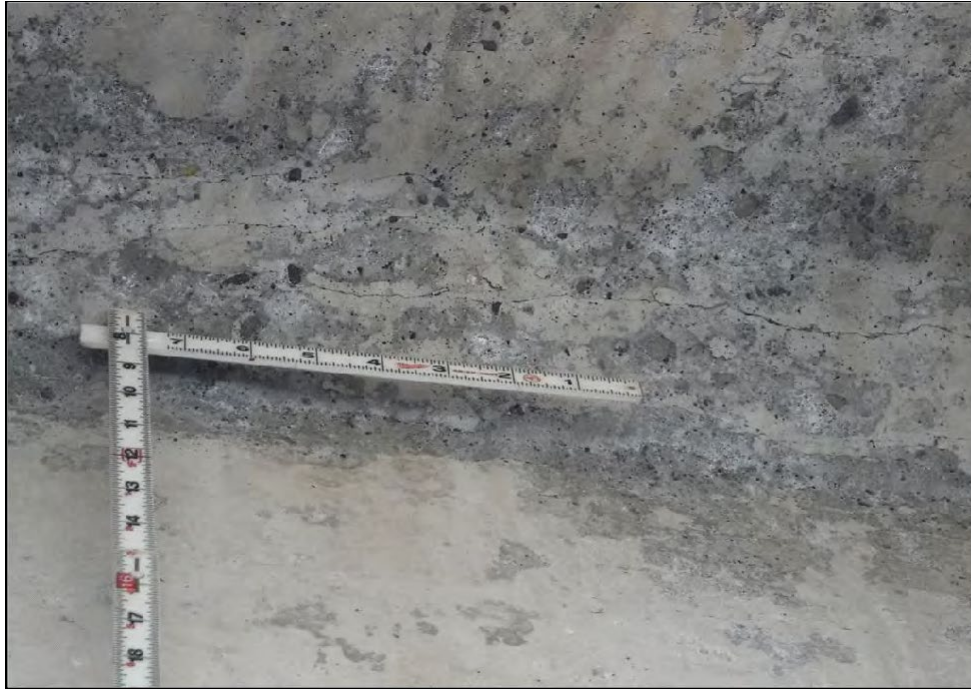
Fillet crack in Girder D near Abutment 2
