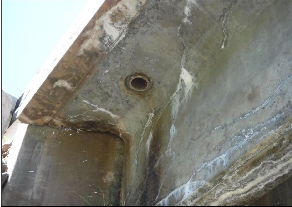
Deck drains not below girder bottom flange
