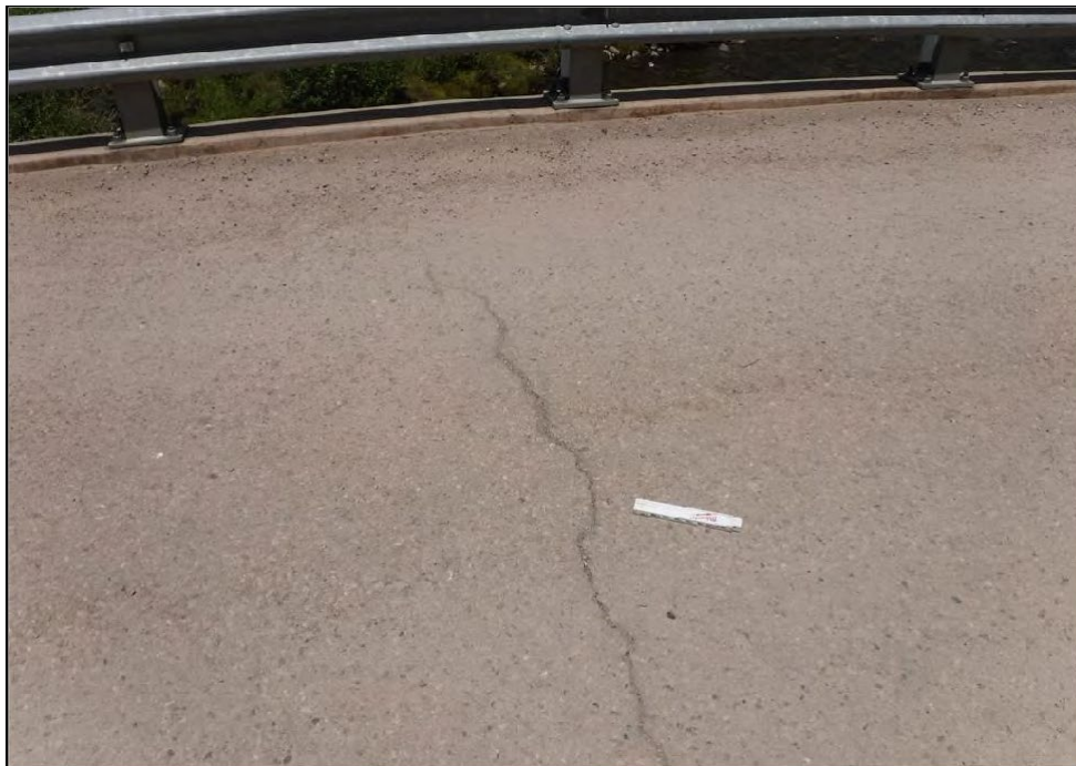
Transverse crack in asphalt on deck
