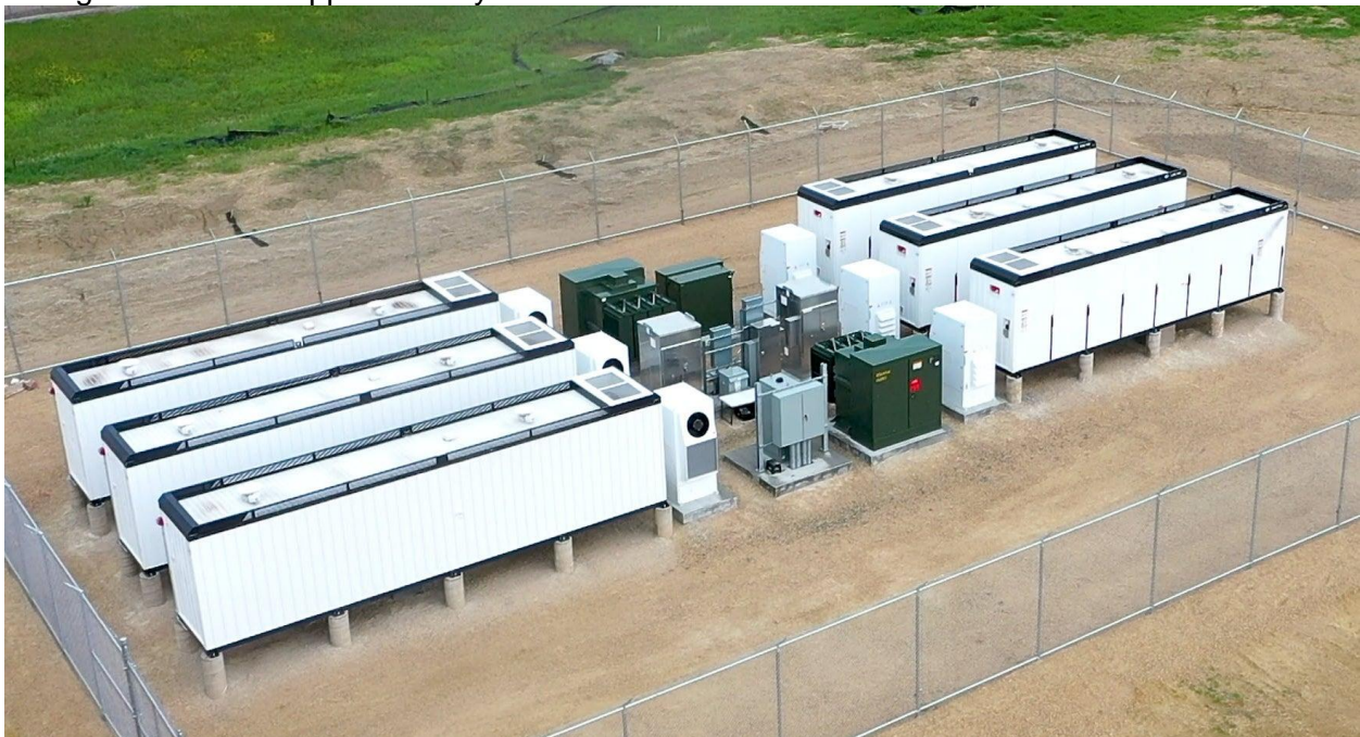
Figure 2. Example BESS microgrid project made of 6 Battery containers, 2 transformers. The Rico Community Microgrid will consist of only 1 Battery Container and 1 Transformer
